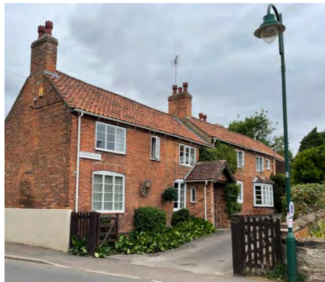
Trackway / Yard - Woodborough
