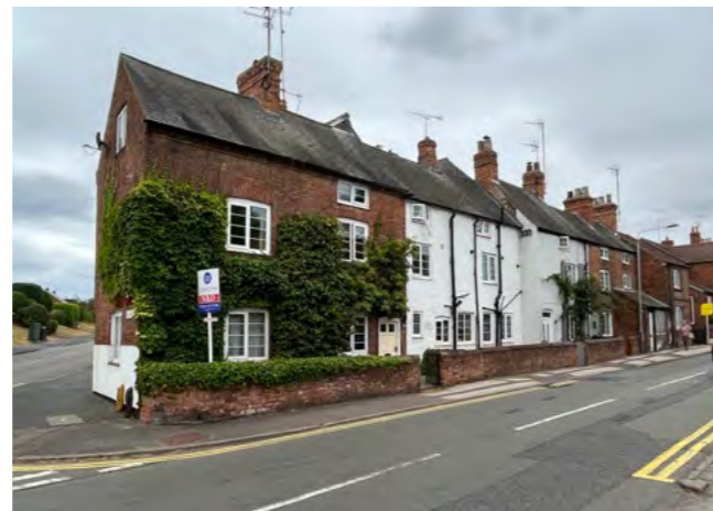
3 storey frameknitter's workshop with windows lining up
