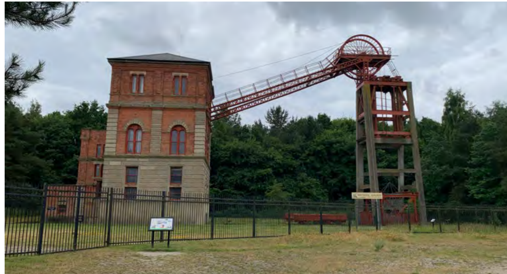
Bestwood Winding Engine House
