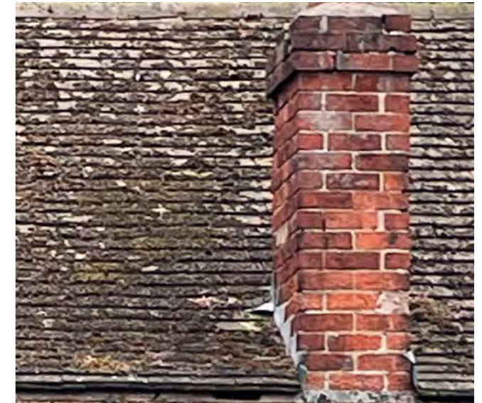
Limestone roof tiles
