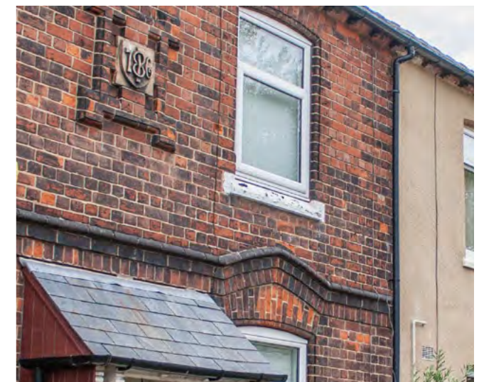
Canopy, corbelling and crest detail
