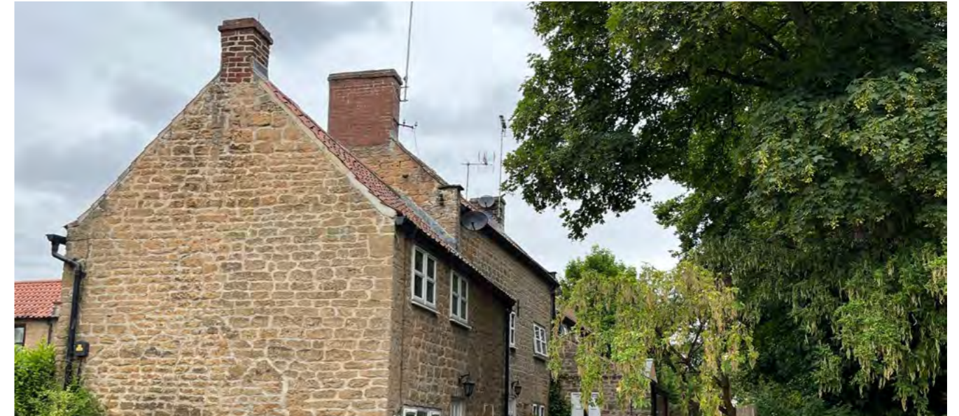
Gable to street with side access, homes running in line with varying heights
