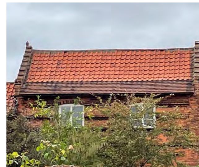
Red keuper marl brick. Roof with 'S' shaped and flat clay tiles.
