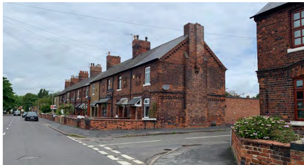
Consistent street line, materials and detailing
