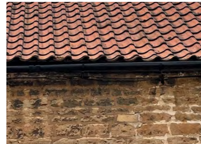
Typical clay pantiles over limestone walls
