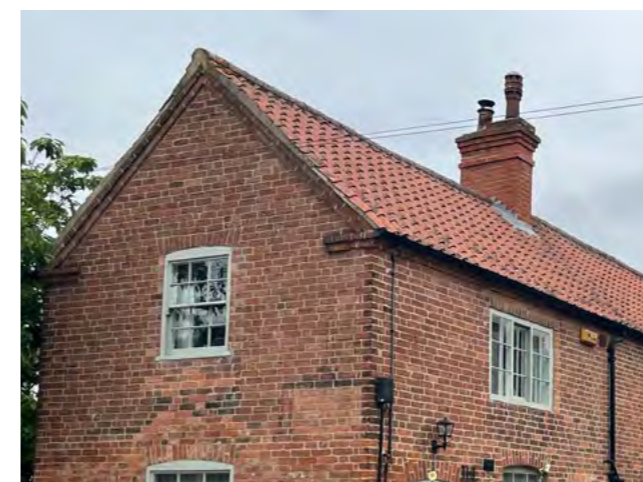
Stepped bricks beneath eaves
