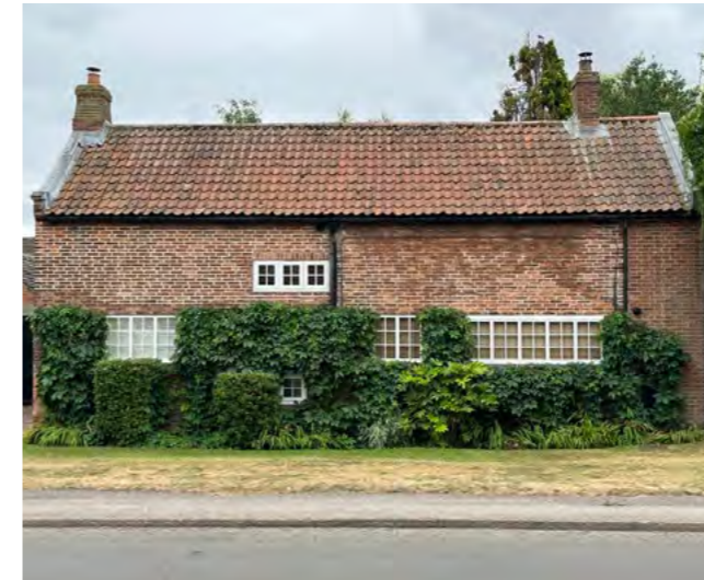
Simple long form and detailing of former barn
