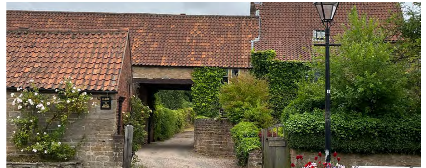
Oversailing roof to farm yard entrance
