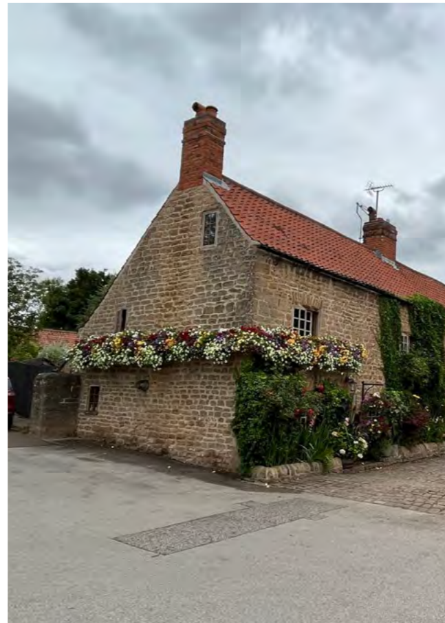
2-storey flat fronted limestone terrace with asymmetric clay tile roof
