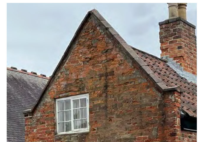
Gables with parapets and simple window
